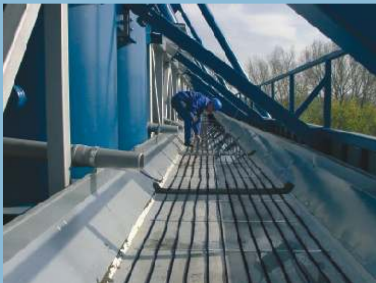
Example of installation of heating cables in roof runner
